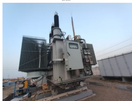
SFSZ-40000/115 Uzbekistan Jizzakh Substation
